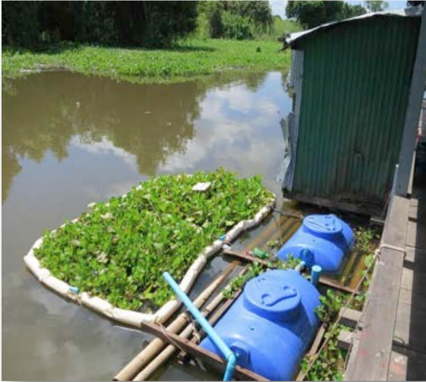
Larger HandyPod system, complete with final-stage hyacinth pond, at a floating school
