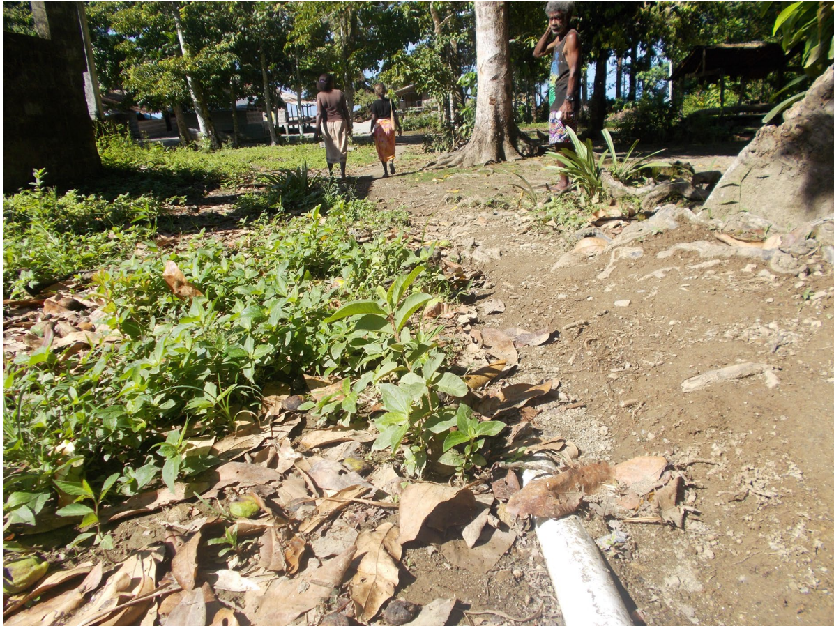
Burying of pipelines – Isunavara community.
