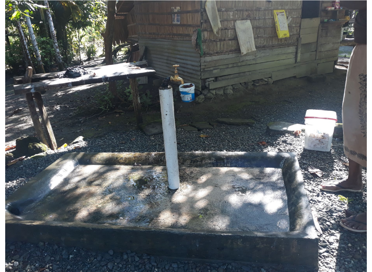
Modified tap to cater for the low water pressure – Isunavara community
