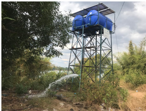
Rehabilitation of Rural Water Supplies
