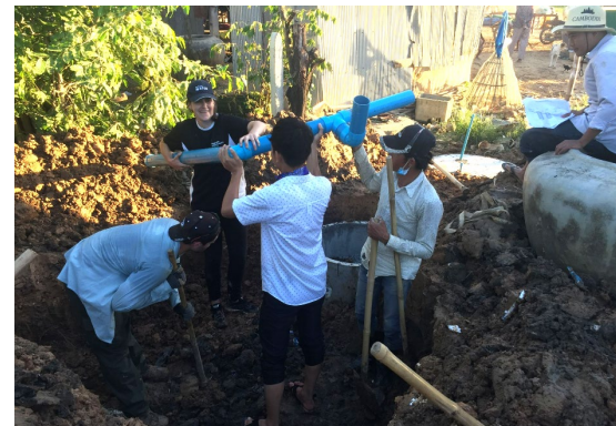
All Seasons Upgrade of Household Pit Latrines
