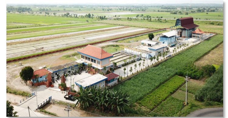
MOJOLAMONG WATER SUPPLY SYSTEM Optimization of Water Supply System
