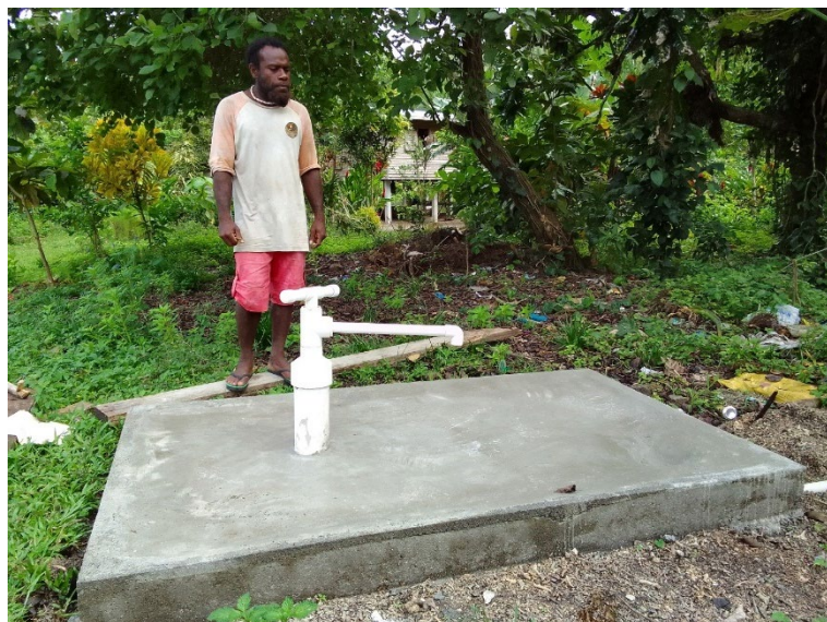
Borehole - Satona community
