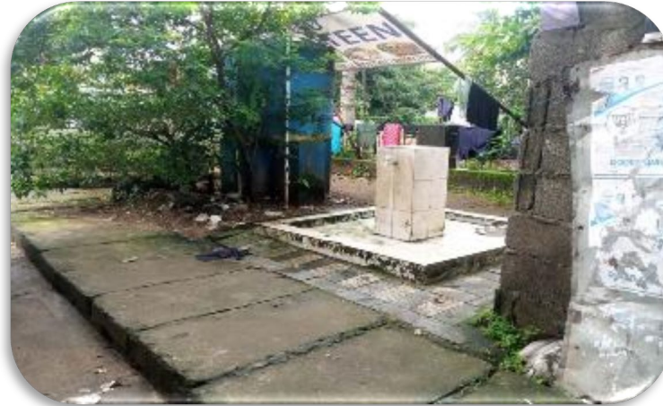
Drain covered with slab
