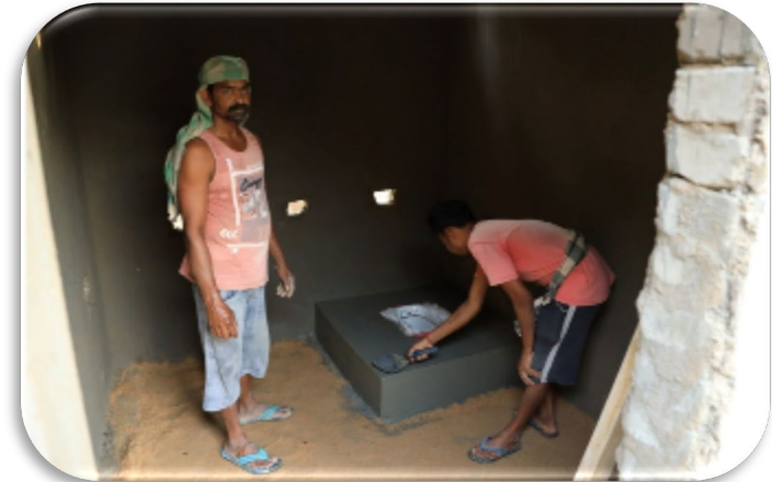
Toilet being constructed
